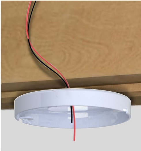
Step 1- Attach Pancake Box to structure Run wires through pancake box (Note: must be home run from remote driver)
